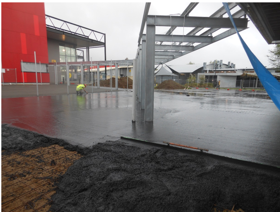
The second concrete pour underway, we were very lucky with the weather that day because it rained just after the concrete had set enough to handle it!
