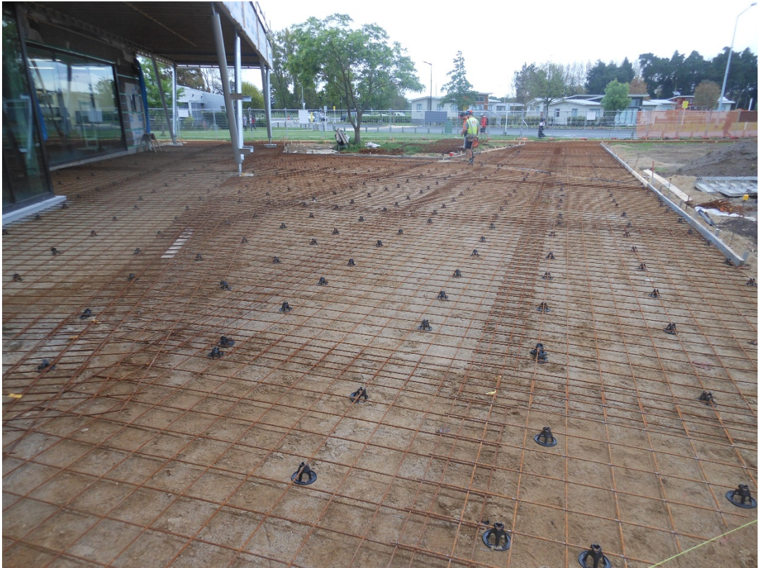
The western entry construction well underway.
