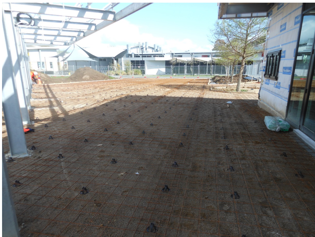
The reinforcing mesh installed ready for some fine weather to pour the concrete.
