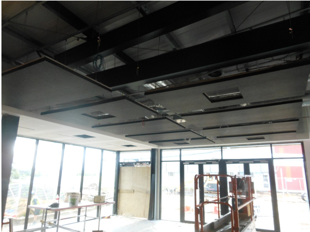
The acoustic ceiling panels being installed inside the new café.
