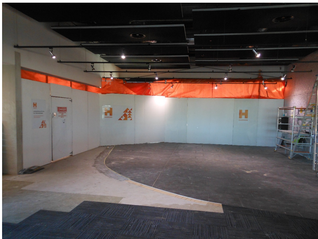
The eastern extension has been hoarded off so there is no chance of dust making it's way out to the café or study space computers.
