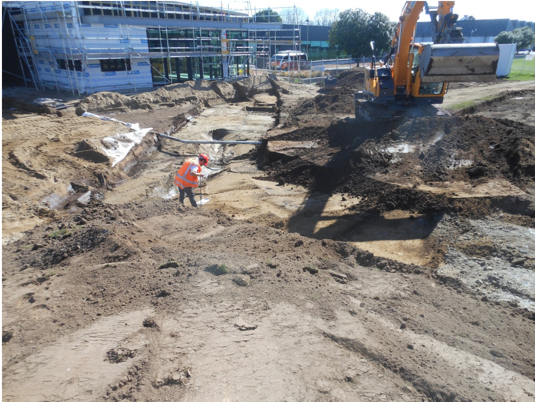
The eastern site works underway, here our engineer is testing the soil in the walkway areas to make sure we removed all the un-suitable fill before we back filled
