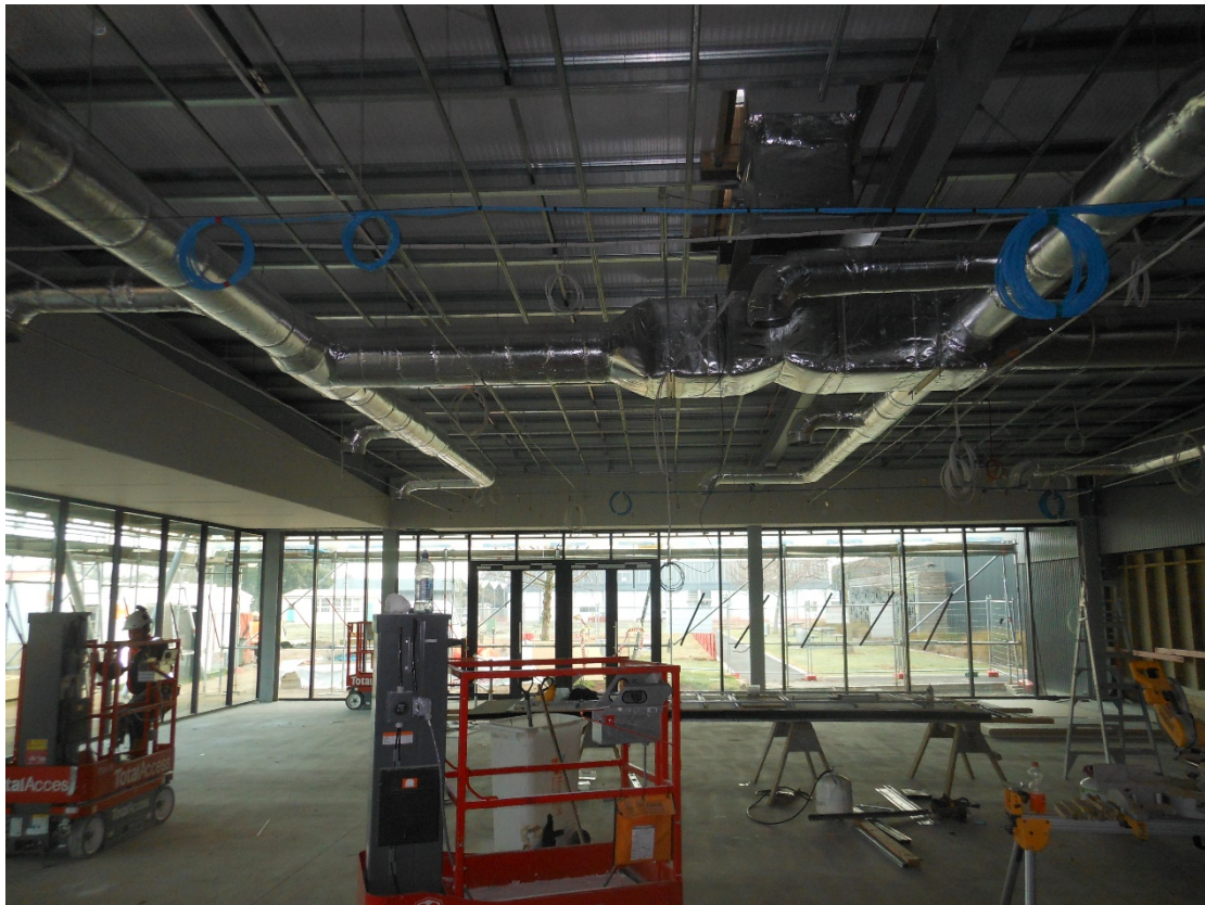
The services are completed and the plaster board is being installed in the western space
