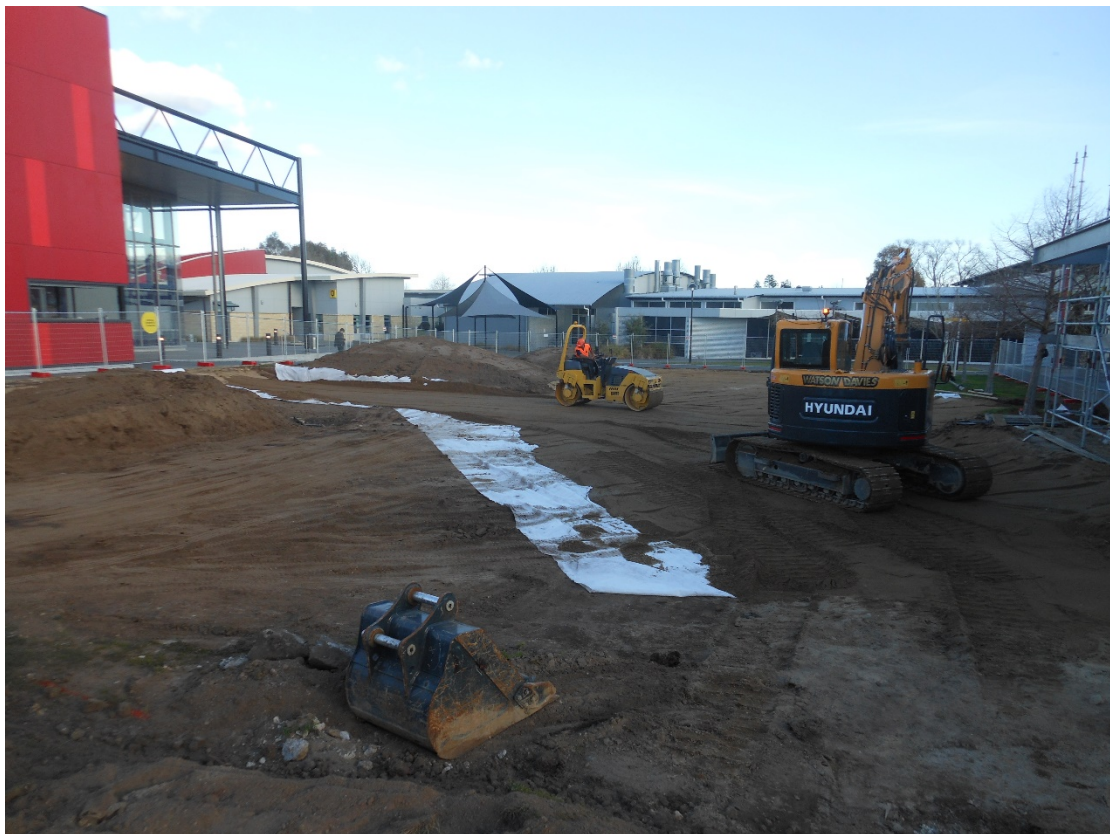
The hard fill being compacted into place for the walkway foundations and footpath areas.
