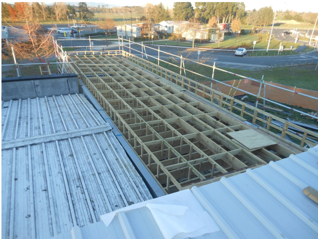
The framing in the western walkway roof was a huge task with approx. 2 thousand metres of timber to be installed at height.
