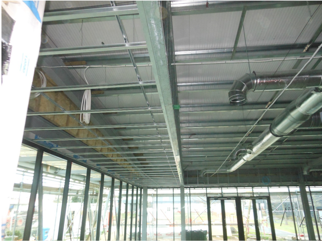
The framing for the bulkhead in the western extension
