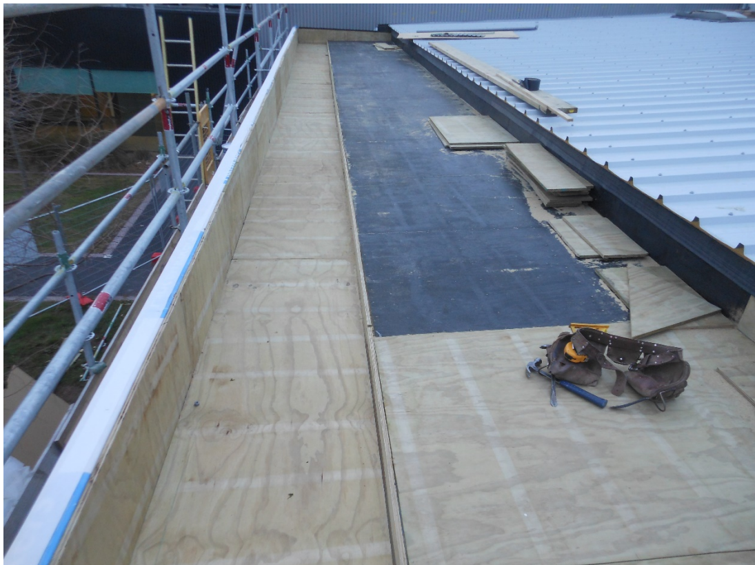
The plywood is well underway on the western walkway roof.
