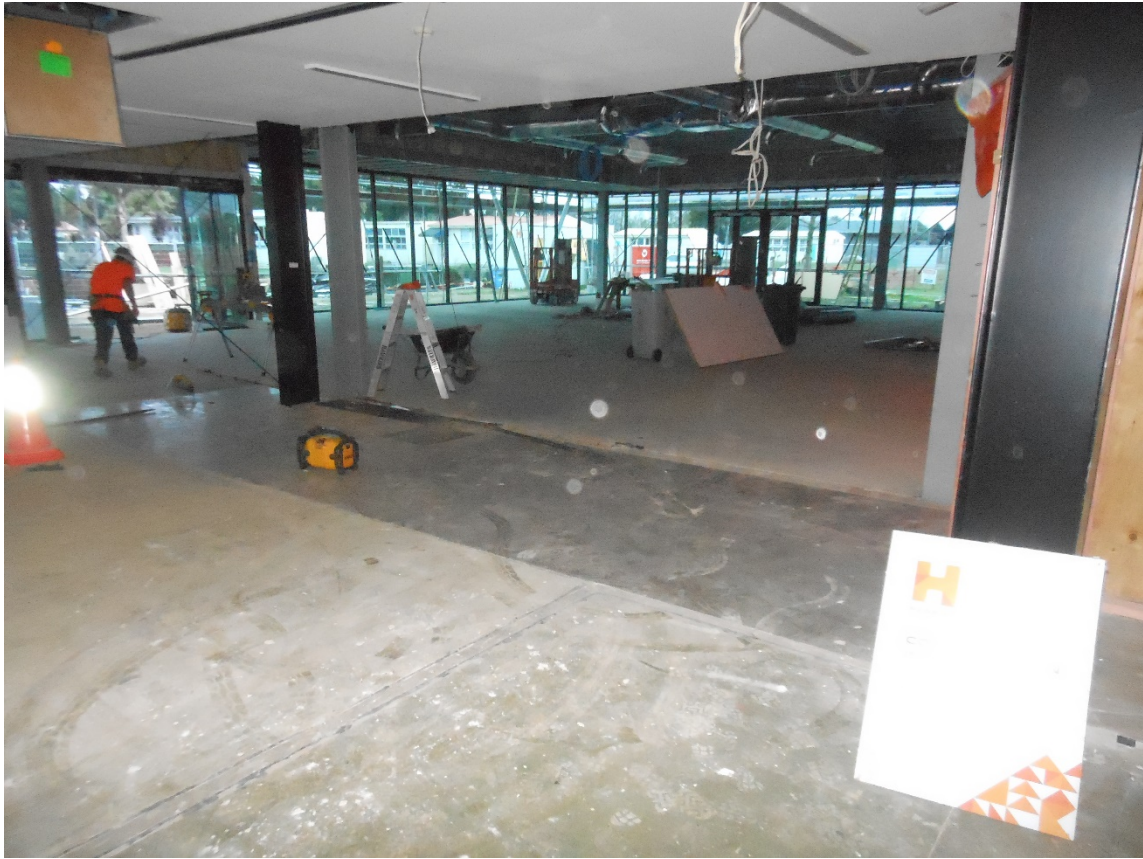
The exterior walls have been removed from the western extension
