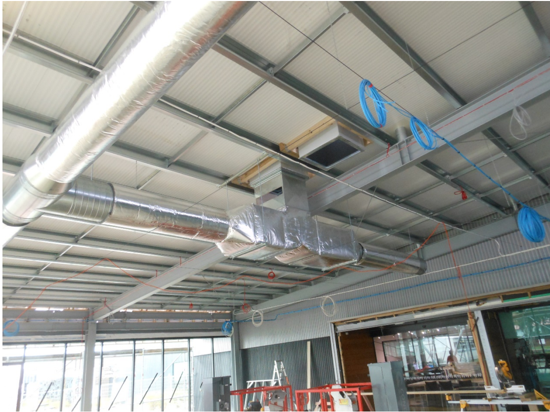
The duct work has been installed through the roof and into the western space
