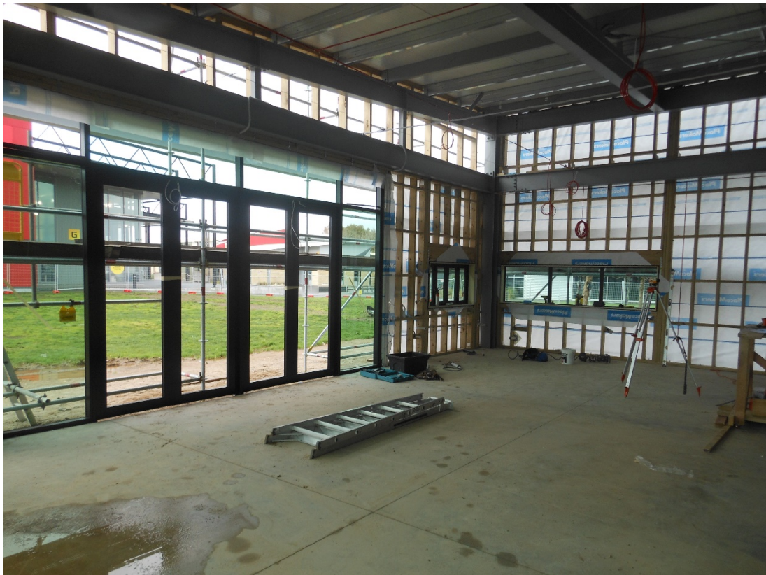
The eastern extension has the new doors and windows installed and glazed.
