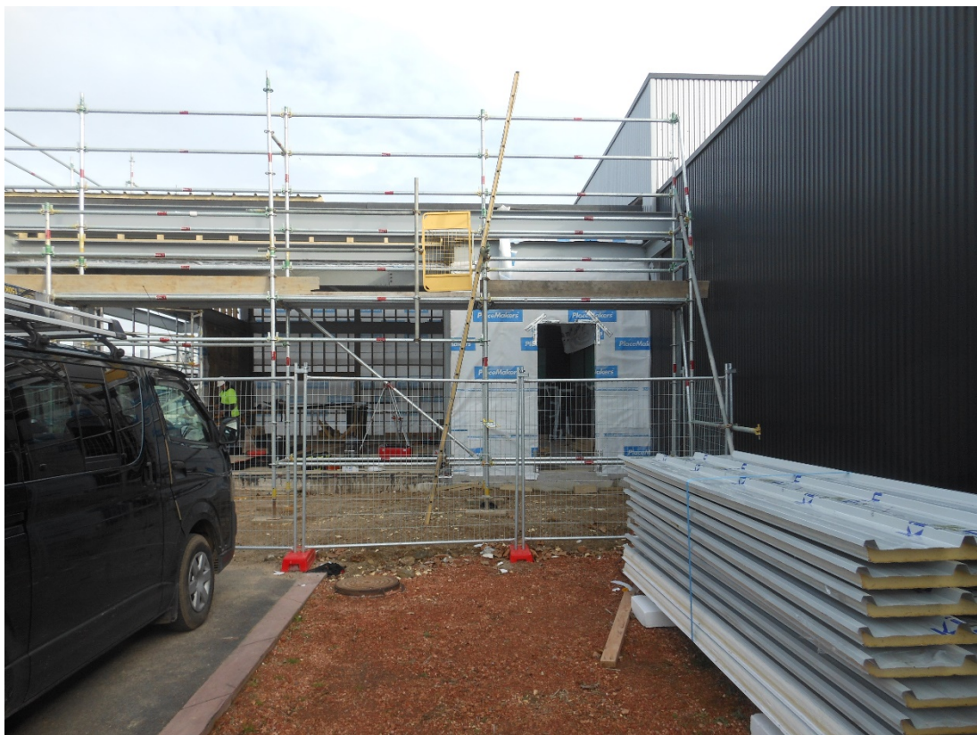
The wall framing on the eastern side completed and wrapped ready for the windows.
