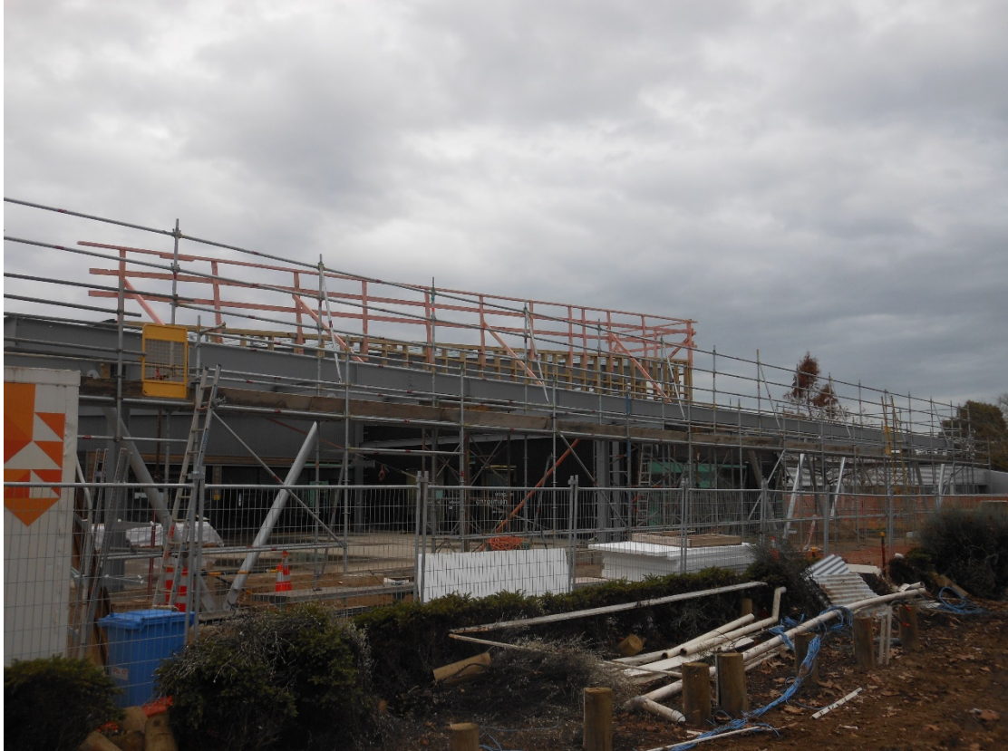
The western side roof edge protection completed
