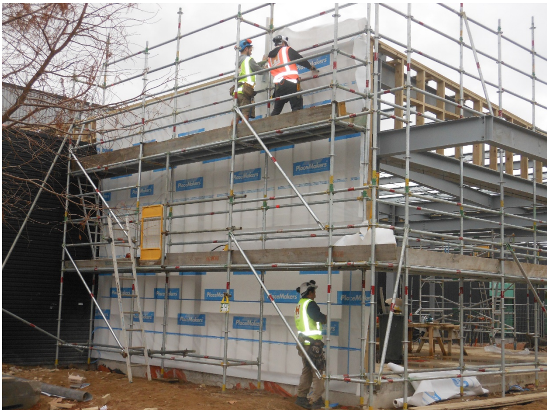
The western side roof edge protection completed
