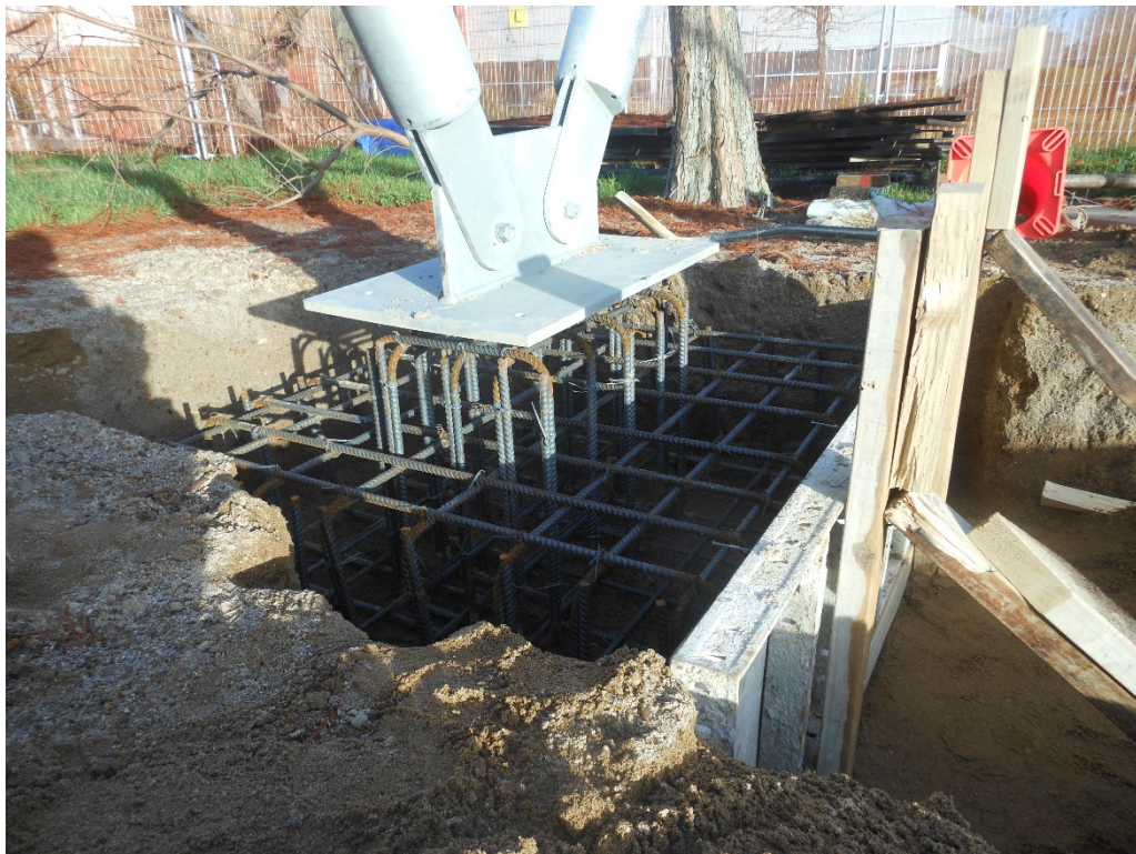
The foundations for the walkway columns have a lot of steel reinforcing in them.
