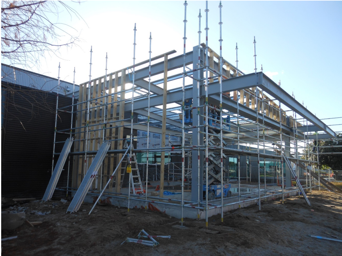
The eastern side structural steel installed and framing well underway
