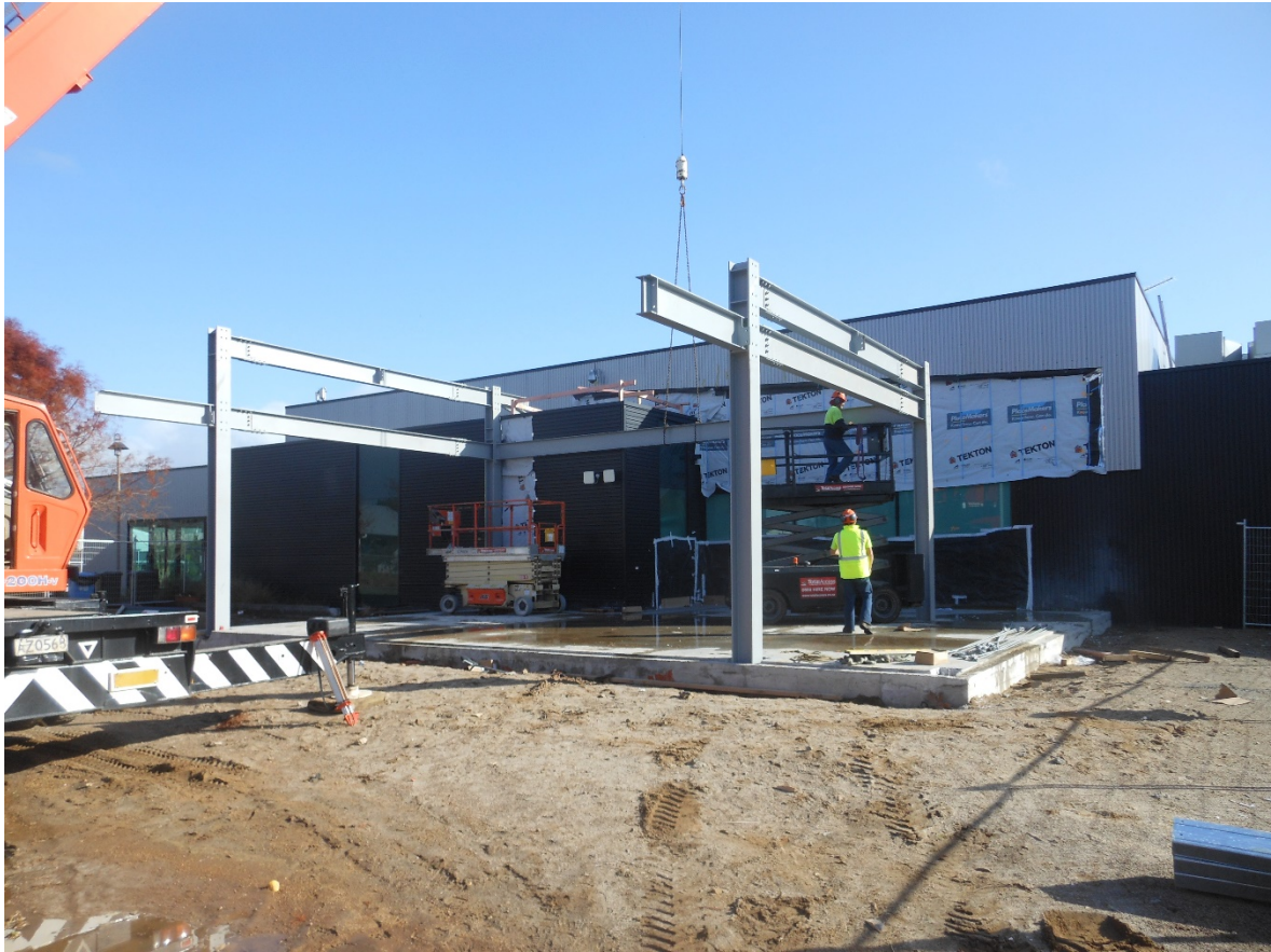
The eastern side structural steel being installed
