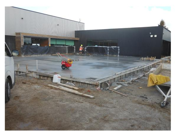
The western slab is receiving a curing compound so there will be no issues with having to wait for it to dry before we lay the floor coverings. Below the eastern slab is ready to pour.
