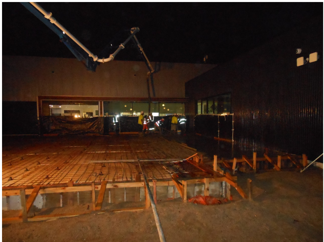
The first floor slab being poured this morning.
