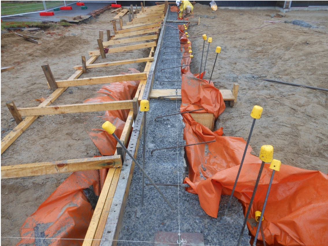
The foundations poured and water blasted so the floor will bind to it.
