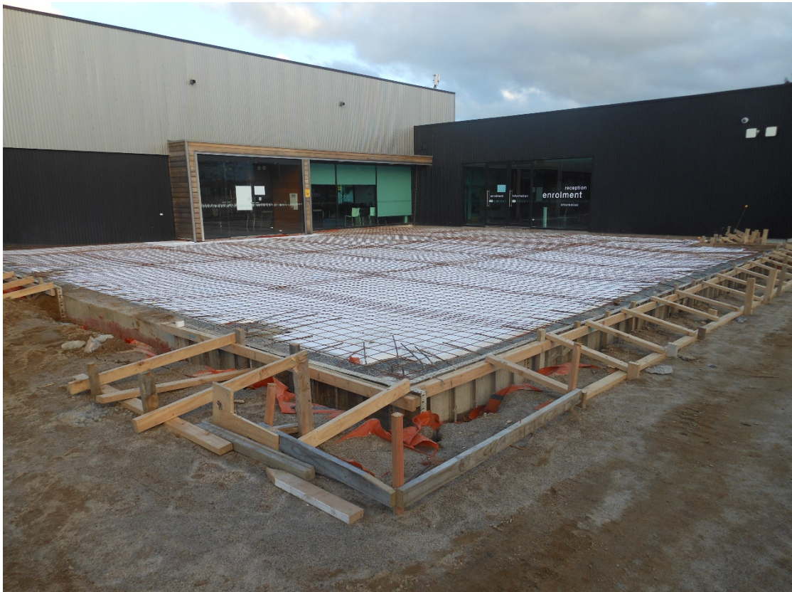
The floor slab is almost ready for the concrete to be poured
