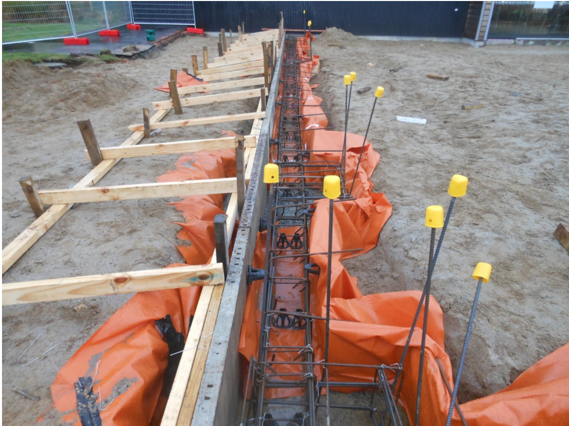
The foundation beams on the western side ready to be poured
