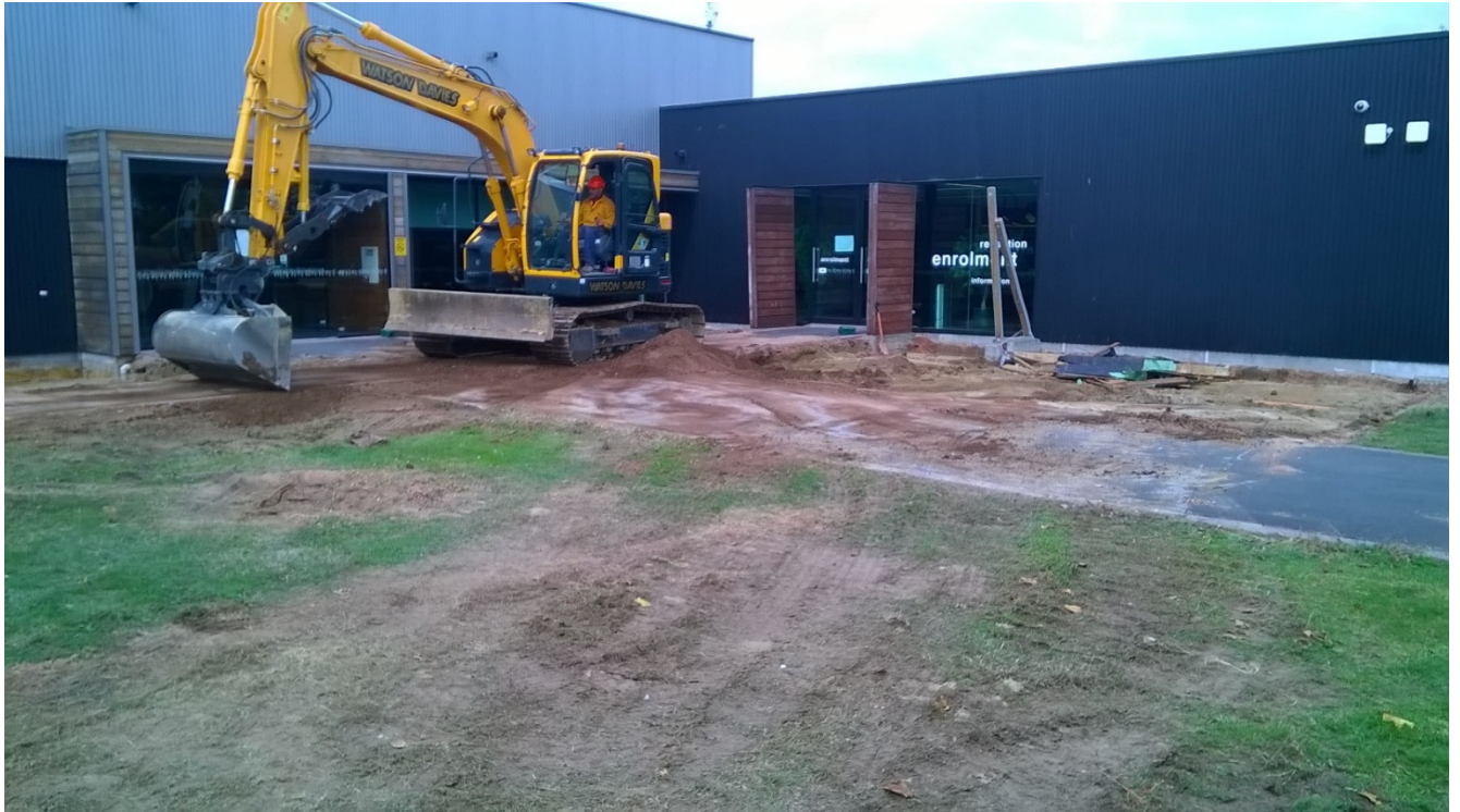
The Excavator is well underway with clearing the site and preparing the ground for the structure
